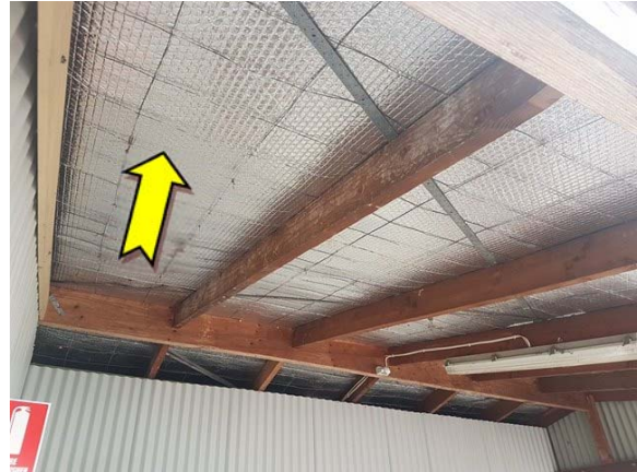
Photo 2. Interior, throughout, underside of roof – suspected SMF sarking insulation material.
