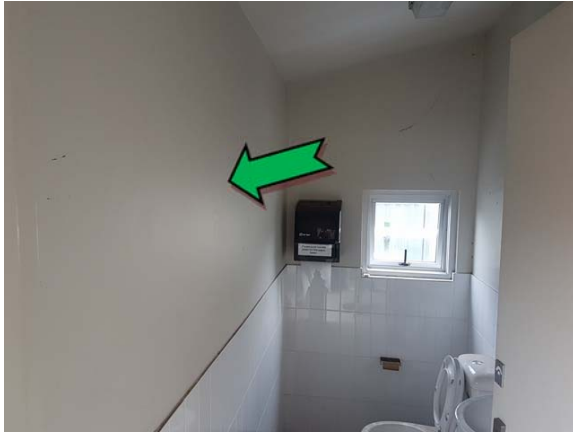
Photo 1. Interior, toilet, throughout, walls – non asbestos-containing fibre cement sheeting.
